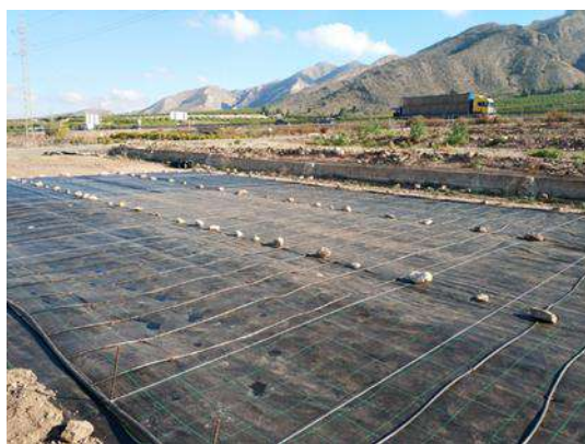
Figure 1.1: Field prepared with anti-weed mesh and hoses installed.
